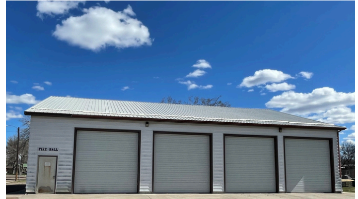
Fort Benton Fire Hall, Fort Benton, Montana
