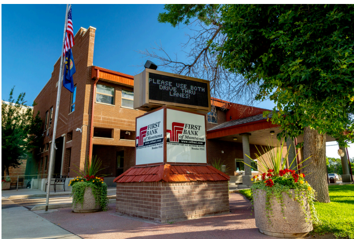
First Bank of Montana, Choteau Branch
